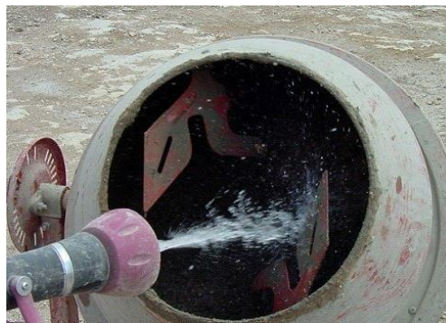
Gambar 2. 3 Penambahan air pada campuran beton (Sumber: https://theconstructor.org/practical-guide/construction-water-qualityspecification/6012/ )
