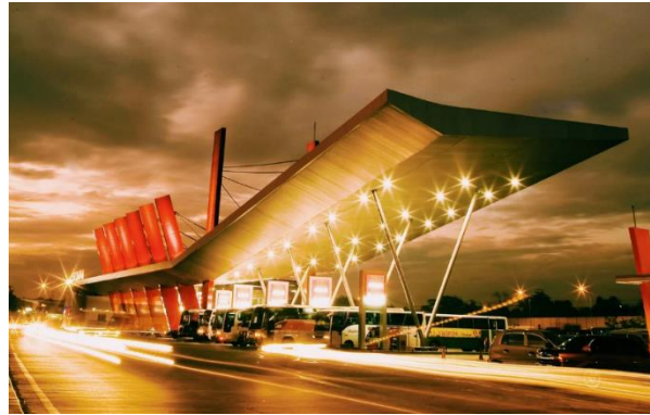
Gambar 2. 21 SPBU Rest Area KM 19 Jakarta-Cikampek
