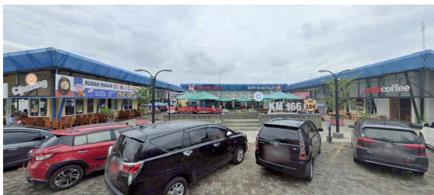
Gambar 2. 30 Pujasera Rest Area KM 166 A Tol Cipali
