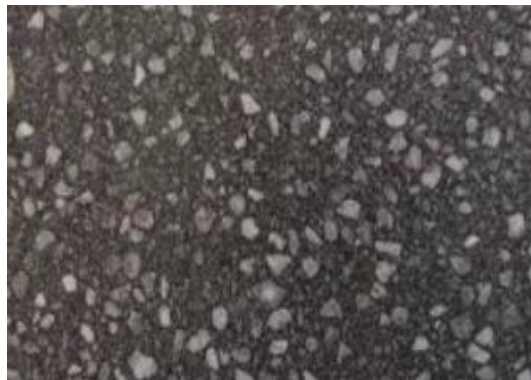
Gambar II. 18 Pengausan ( Polished Aggregate ) Sumber: Dinas PUPR Kab. Kulon Progo
