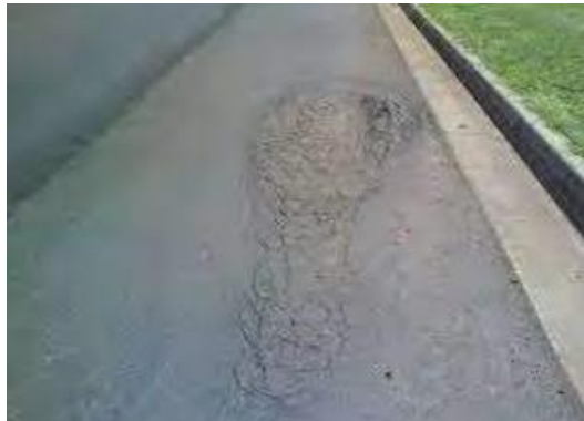
Gambar II. 12 Sungkur ( Shoving ) Sumber: Dinas PUPR Kab. Kulon Progo
