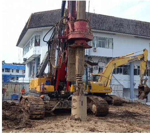
Gambar 2.1 Bore Pile
