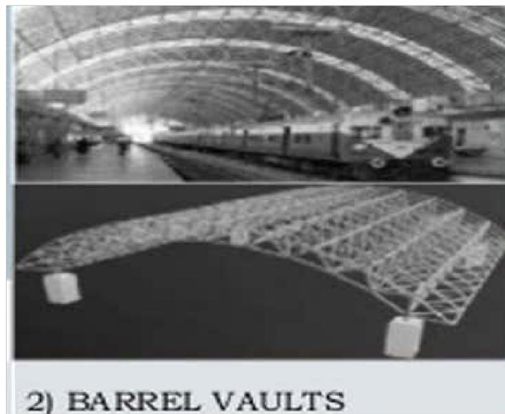
Gambar 2.14. Barrel Vaults
