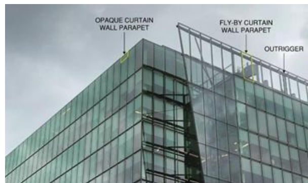
Gambar 5.12 Contoh Cutarin Wall Jenis Unitized
