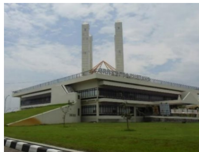
Gambar 2.18 View entrance PERPUSDA Grahatama Pustaka
