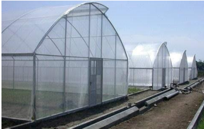
Gambar 2. 28 Greenhouse tipe Tunnel
