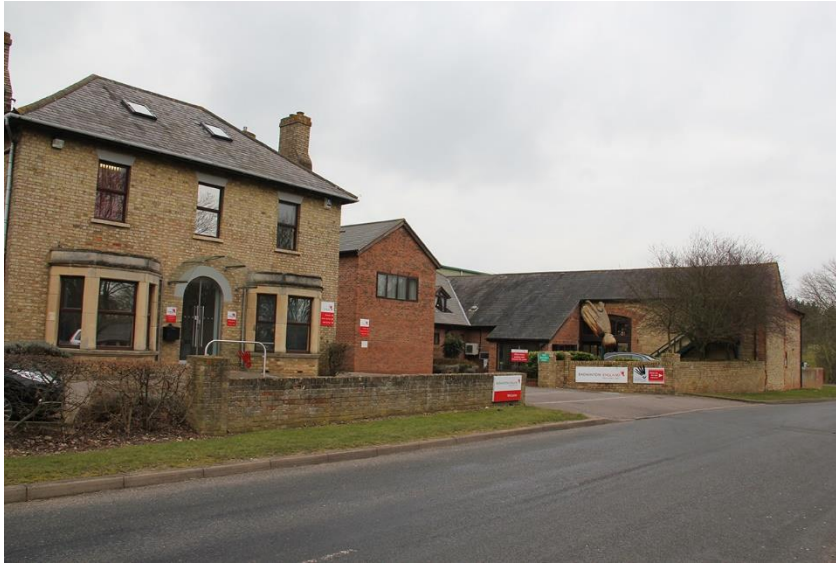
Gambar Bangunan National Badminton Museum Milton Keynes
