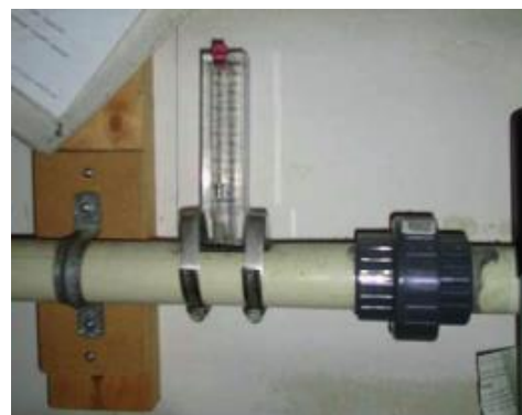
Gambar 2.13: Flow Meter Sumber: google image
