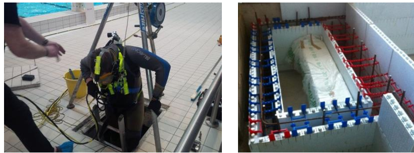
Gambar 2.9: Balancing tank Sumber: google image
