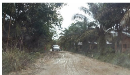
Gambar II.16 Akses jalan di Teluk Jering Sumber : https://journeysn.wordpress.com/2018/11/02/jalan-jalan-ke-wisata-teluk-jering/
