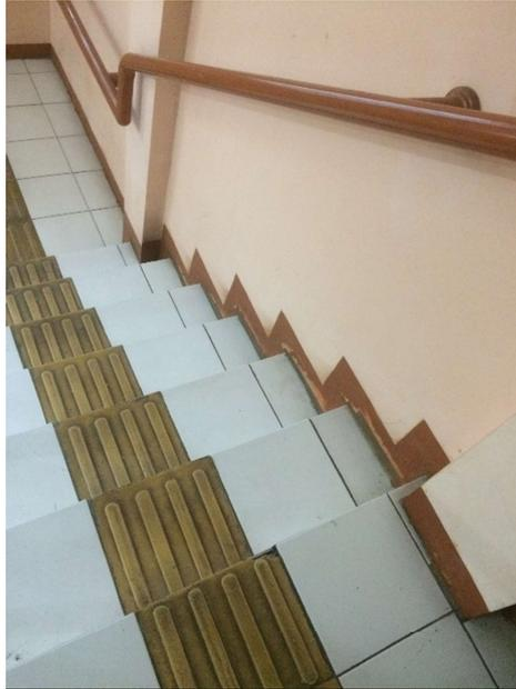
*Gambar 2.15 Jarak Railing Tangan dan Guiding Block*
