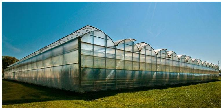
Gambar 4.2 Konstruksi ridge and furrow
