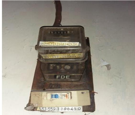
**Gambar 2.4 KWH meter analog**
