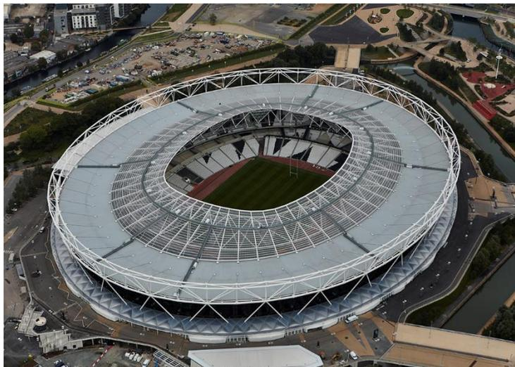
Gambar : 3.5 Tension Ring Structure
